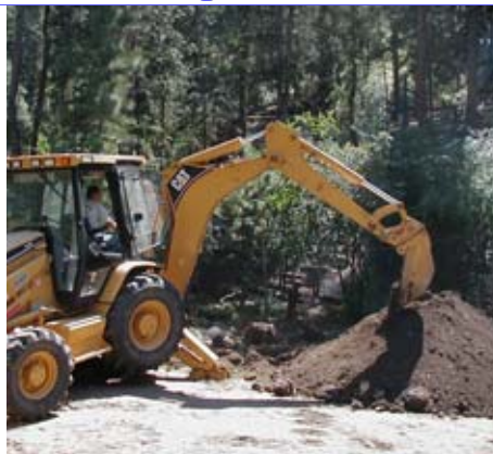
Brad from Lockman Excavating
