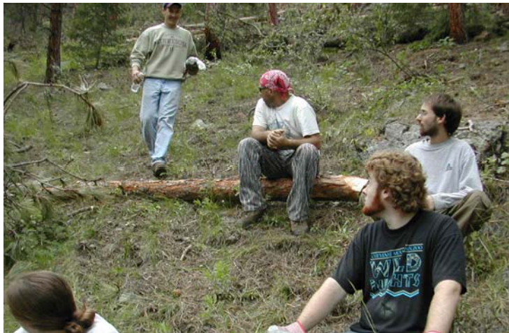
Jesse & crew taking a break while building fence.
