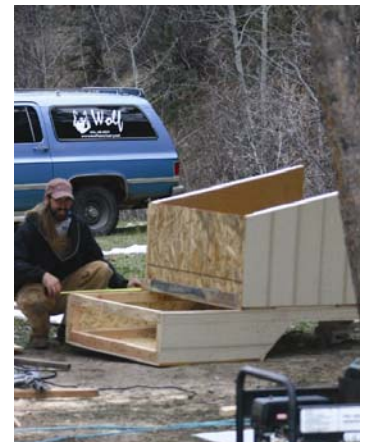
Building a heated dog house.
